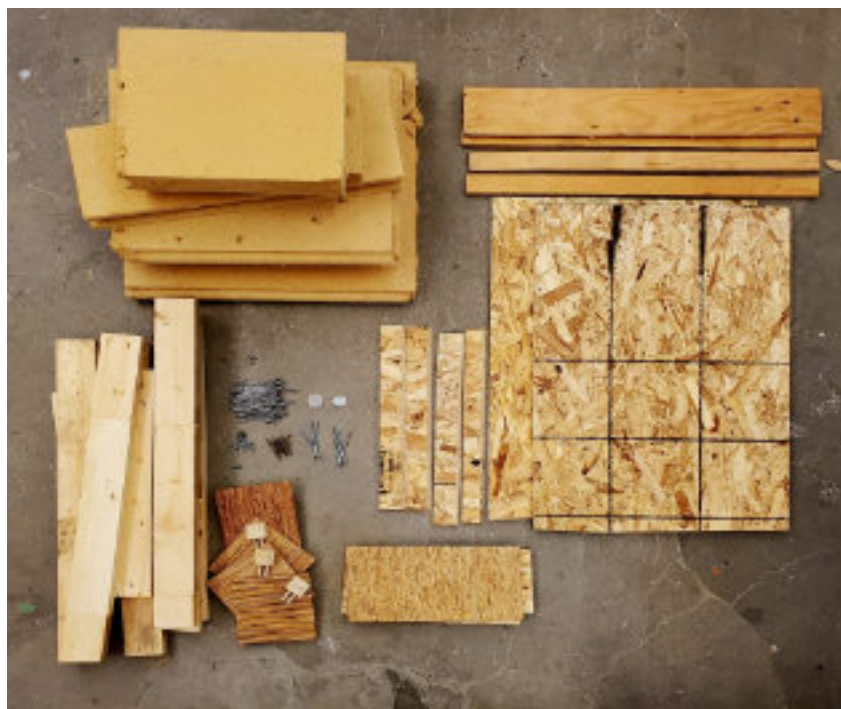
Figure 53 Wall mock-up in deconstructed form, credit Kaia Nielsen_Roine, image source: https://blogs.ubc.ca/design4deconstruction/designfordeconstruction/
