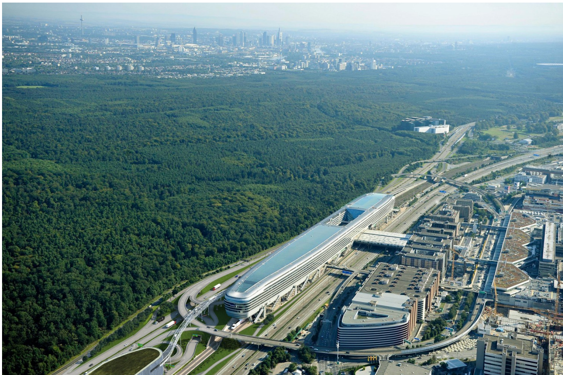
Rys. 9. Widok na Airport City we Frankfurcie (Archdaily, 2021)
