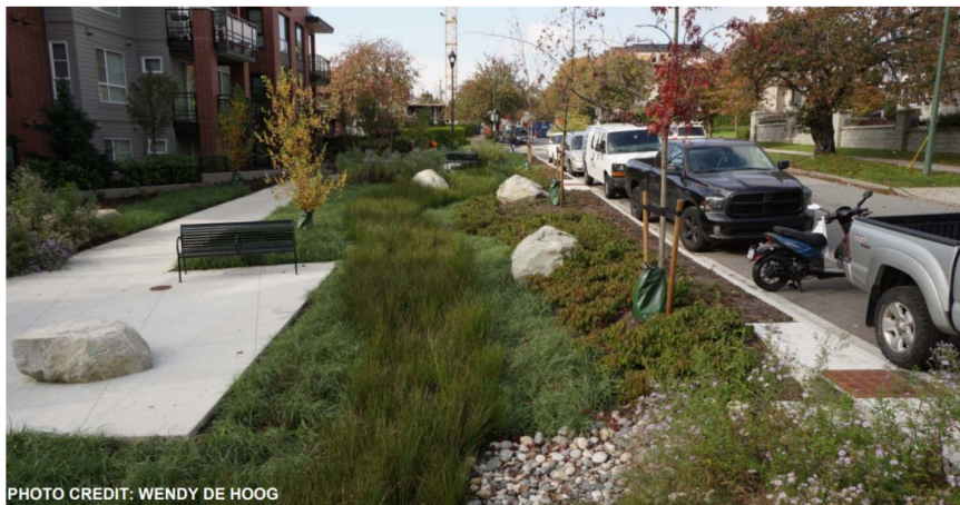
Figure: Bioretention installation at Yukon Street and 63rd Avenue, Vancouver
