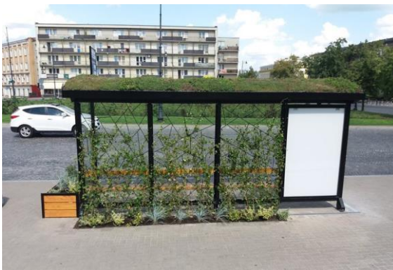
Figure 4.4. Intensive green roof in Warsaw. Source: FPP Eviro, Białystok City Office, https://www.lifetreecheck.eu/en/Databaze/2019/Green-Bus-Stops
