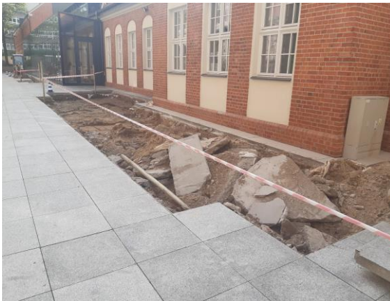
Figure 5.8. The public space in September 2022. Own photo
