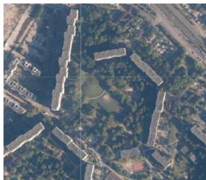
Fig.14.9. Example buildings for PV installation, source: https://mapy.geoportal.gov.pl/
