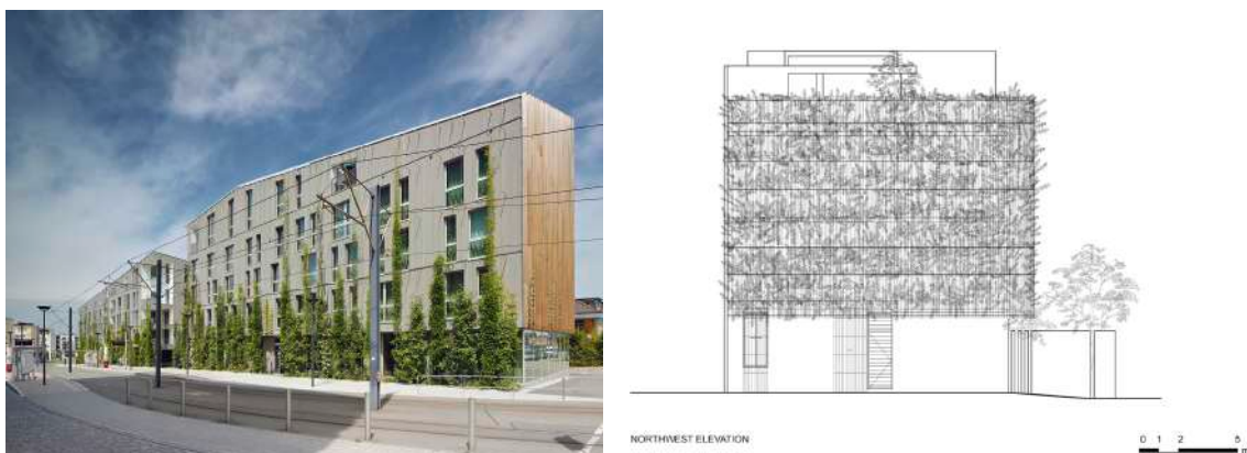
Fig.14.3. Stadthaus M1, Freiburg using rope system (left), steel structure connected to the elevation (right) source: GreenSolutions Catalogue by Jakob Rope Systems,
