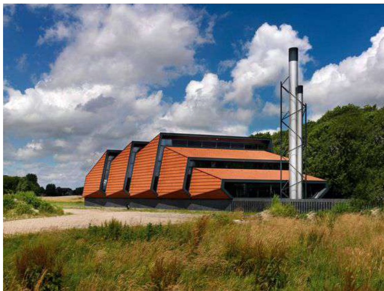
Fig.14.6. Eco Zathe combined heat and power plant, photo by Gerard van Beek.
