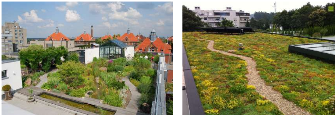
Fig.14.4. Intensive green roof in Germany (left), https://efb-greenroof.eu/work/intensive-green-roof-germany-4/ , extensive green roof in Portugal (right), https://efb-greenroof.eu/work/extensive-green-roof-portugal/ .
